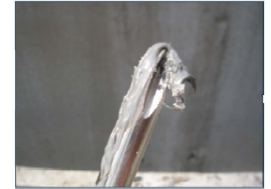
Wet epoxy component extracted from bridge hole 200
